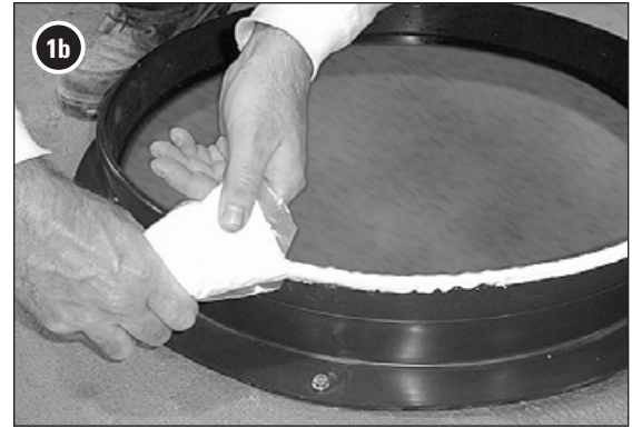
MA320 adhesive on bolt-down riser lid adapter
