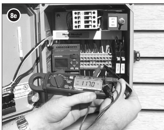
Measuring dynamic pump voltage
