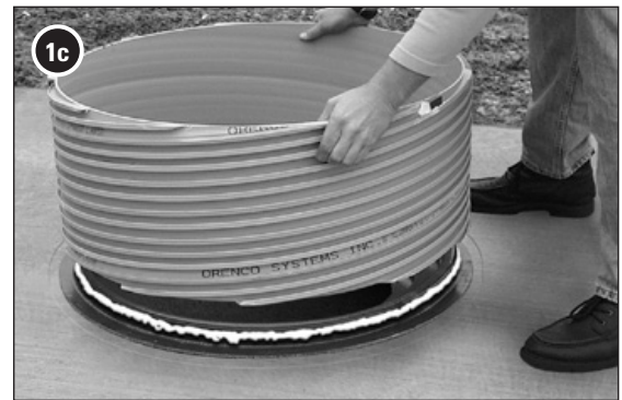
MA320 adhesive on bolt-down riser lid adapter
